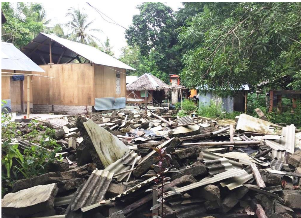
Figure 1. Debris caused by the Lombok Earthquake (2018) showed many broken asbestos roofing (Source: Shelter Cluster Indonesia)
