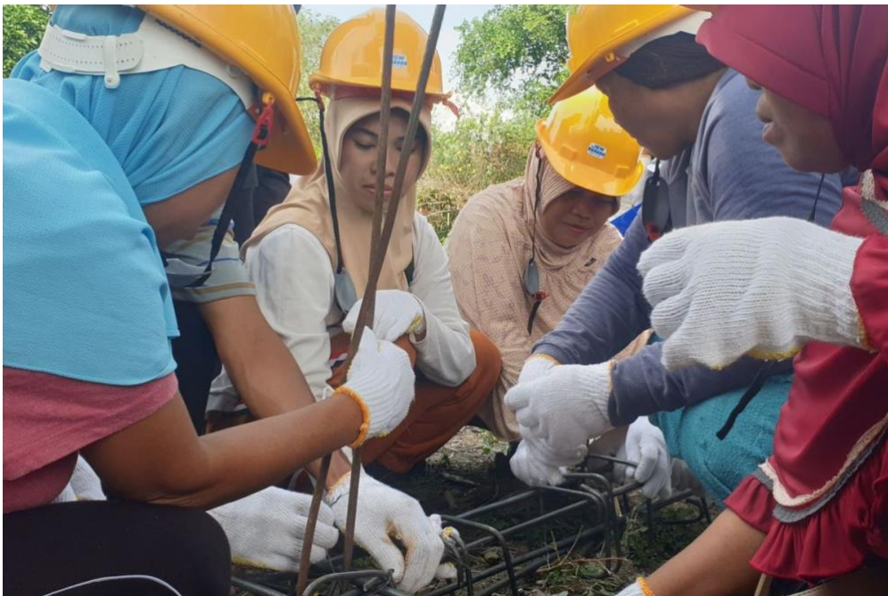
Figure 1. Women groups were trained to learn about housing reconstruction in Central Sulawesi (Source: Kompas)
